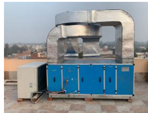
Air Handling Unit (AHU)
